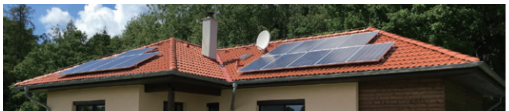
▼ ENERGY STORAGE SYSTEM
